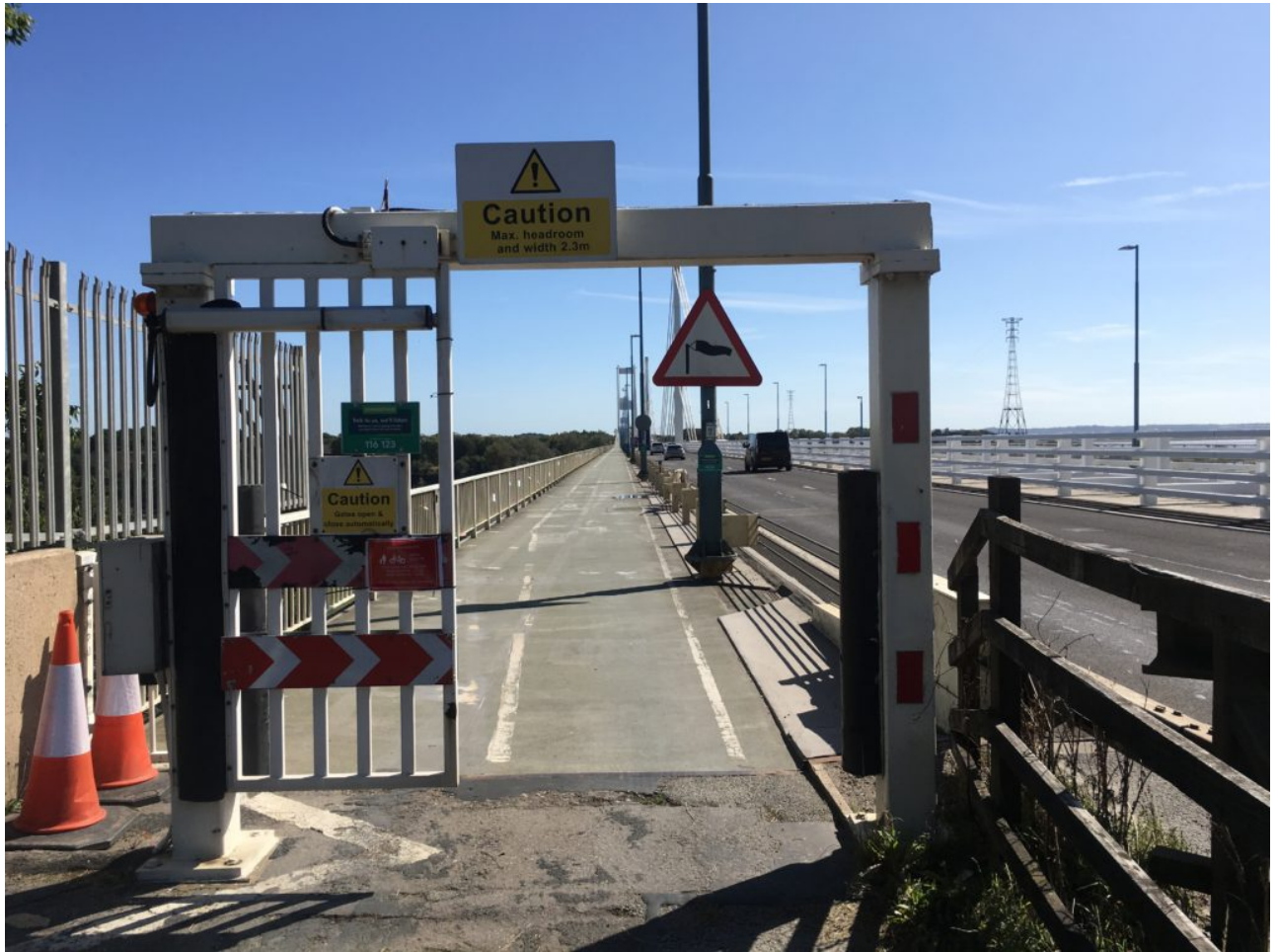
Old Severn Crossing automatic gate
