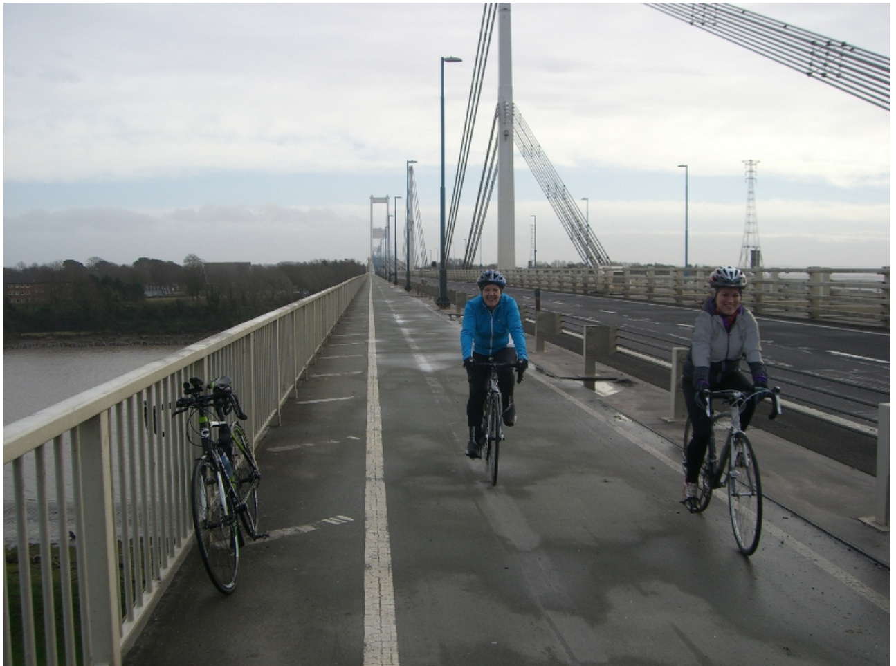
Old Severn Bridge, cycle and walkway
