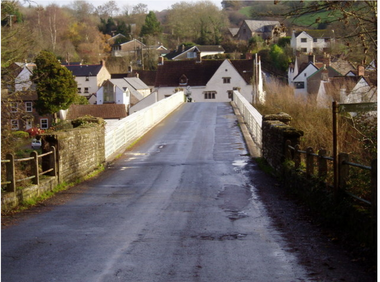
Brockweir Bridge crossing from Wales to England near Tintern
